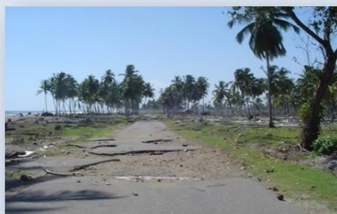
Road damaged by the tsunami in Aceh, Indonesia
